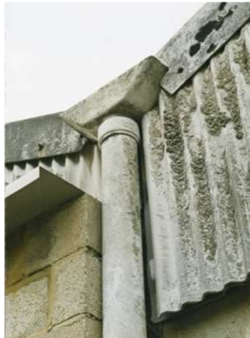
Asbestos cement downpipe, hopper and profile sheet
