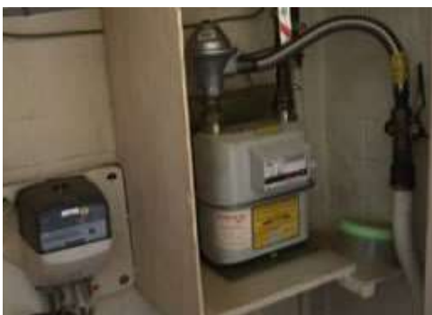
Asbestos panelling around a gas meter
