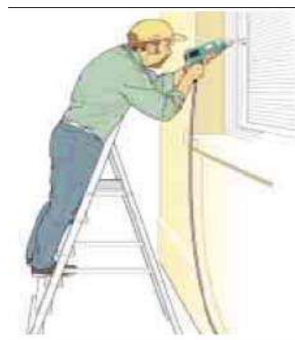
Correct – steps facing work activity
