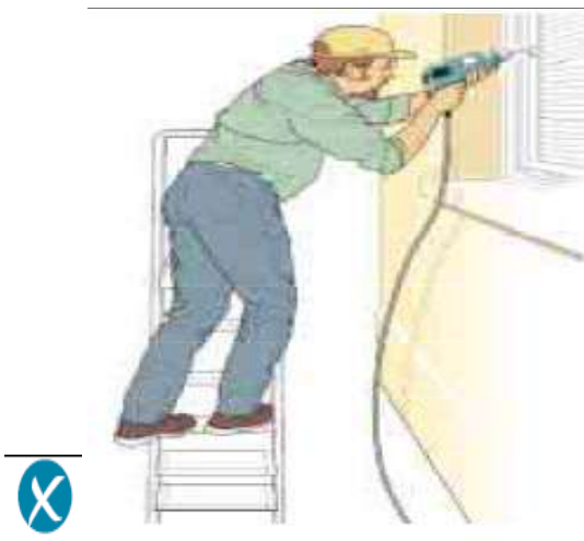
Incorrect – steps side on to work activity
